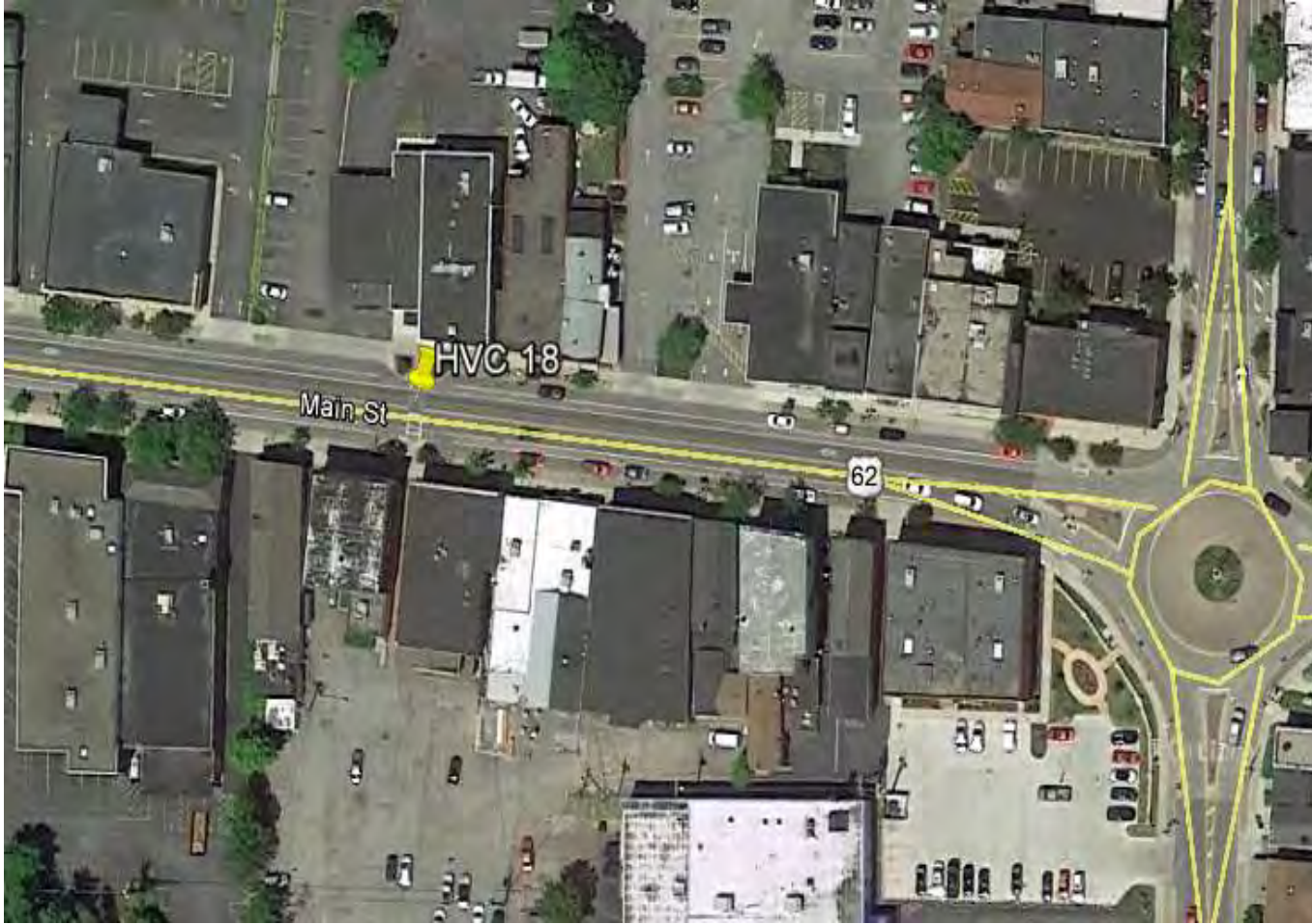
Figure 3.2. Aerial view of HVC location 18 (Main Street) in Hamburg. (Source: Google Earth)
